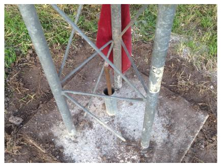
In this installation, the ground rod is equidistant from each tower leg and very close to each. Three ground straps will converge on the same ground rod. There will be a very small angle between the ground straps and the tower legs hopefully taking most of the current down the center but not touching the concrete. Yes, this is not a good example because the concrete base is small, but normally there would be much more concrete. This is a retirement income installation.
